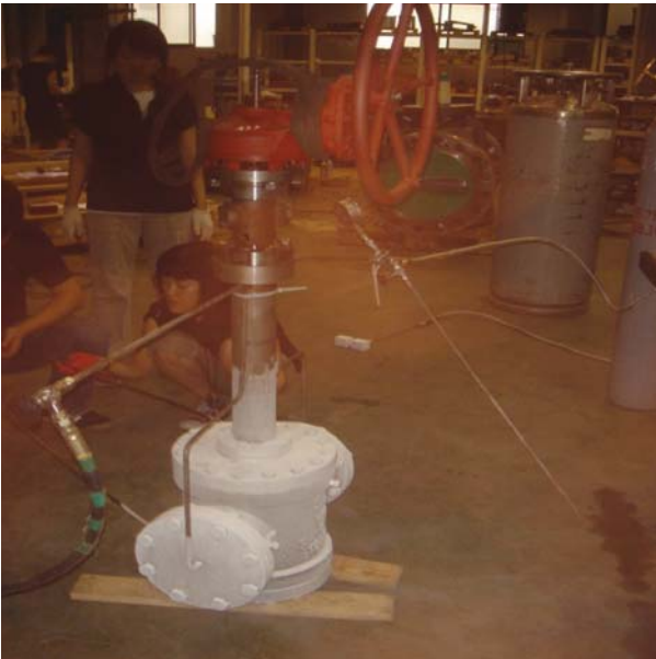
After Cryogenic Test at Factory
